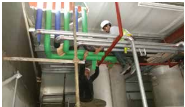
Insulation of Chiller Piping
